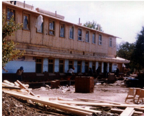
Addition under construction in 1989
